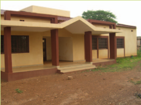
When we visited, the centre was getting ready to move to this new building.
