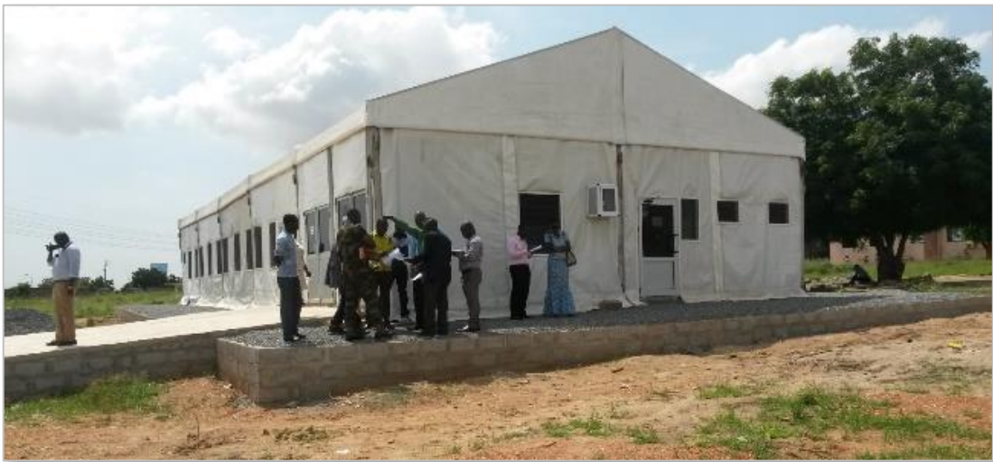
Ebola isolation center construction site at Tema
