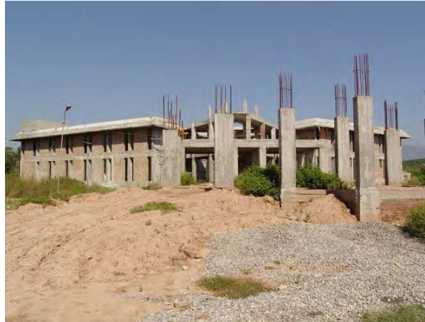
■ Building works underway at the new Health Services Academy campus.
