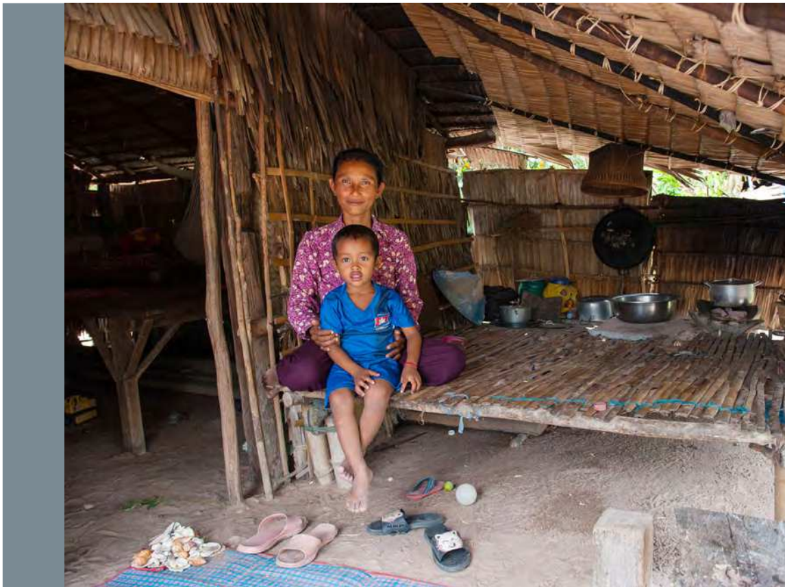
● A traditional rural Khmer house – like this one where Chew Yem lives with her three children – is made of wooden posts and slats, with a raised floor and thatched palm leaf roof and sides, while newer houses may have metal roofs and walls. Observable features such as building materials, size and condition of the house are part of the IDPoor questionnaire.
